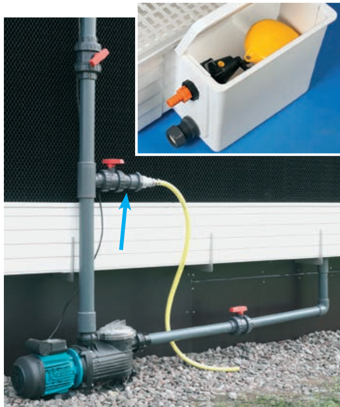
Centrifugal pump incl. filter and bleed-off
