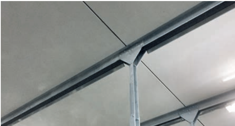
The smooth, white surface of the plastic panels' underside allows fresh air to flow crosswise through the barn without obstructions and also increases brightness in the lower level
