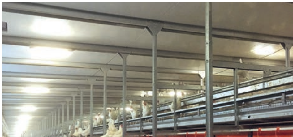
The smooth, white surface of the plastic panels' underside allows fresh air to flow crosswise through the house without obstructions
