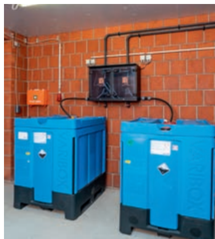
Acid and alkali dosing
