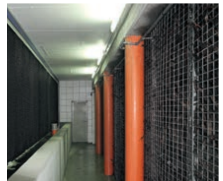
Cleaning stage 3: brushwood filling to transform odorous substances
