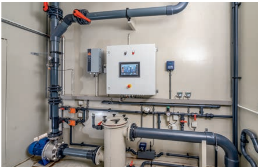
Pre-installed technical room with control box
