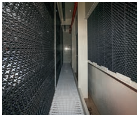
Filter wall (left) and droplet separator (right)
