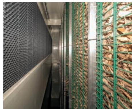
View into the second pressure chamber: droplet separator (left), biological filter wall (right)
