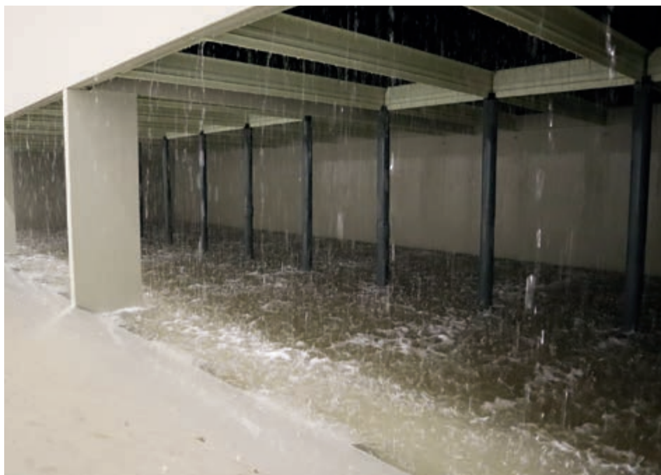
Porcus air scrubber in operation
