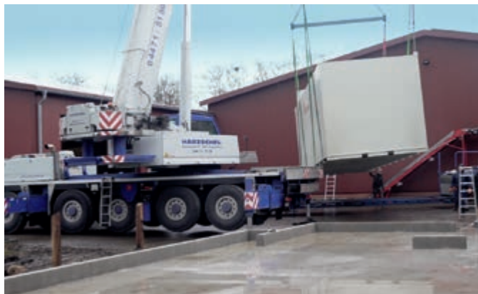
A crane lifts the Porcus air scrubber from the low loader
