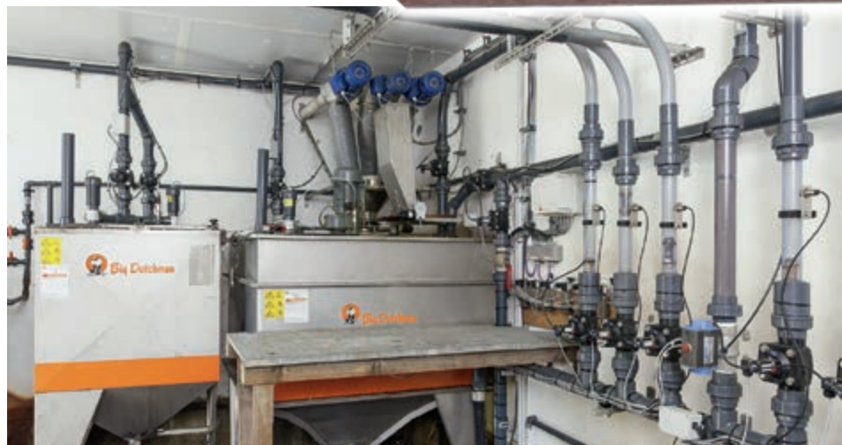
1-tank system with rinse water tank and four JET branch lines
